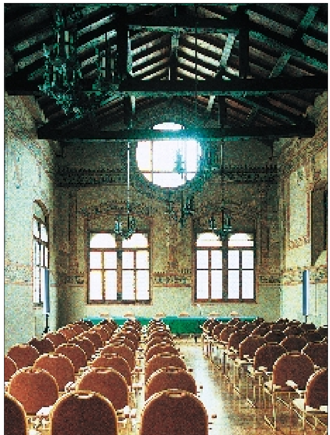
Sound system for conference rooms with reinforcement speakers for the audience area.
